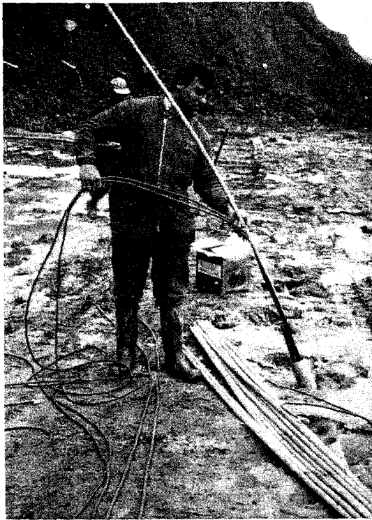
Photo 25.3. The placing of a bottom charge and the high core load cord in a contour blasthole.
