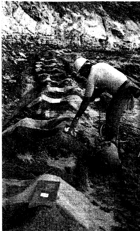
Photo 25.6. Placing a pneumatic plug to produce stemming. (Courtesy of Atlas Powder Co.)
